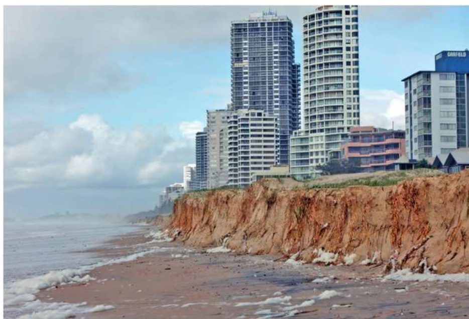
Figure 3.25: Beach erosion at Brisbane, Australia
