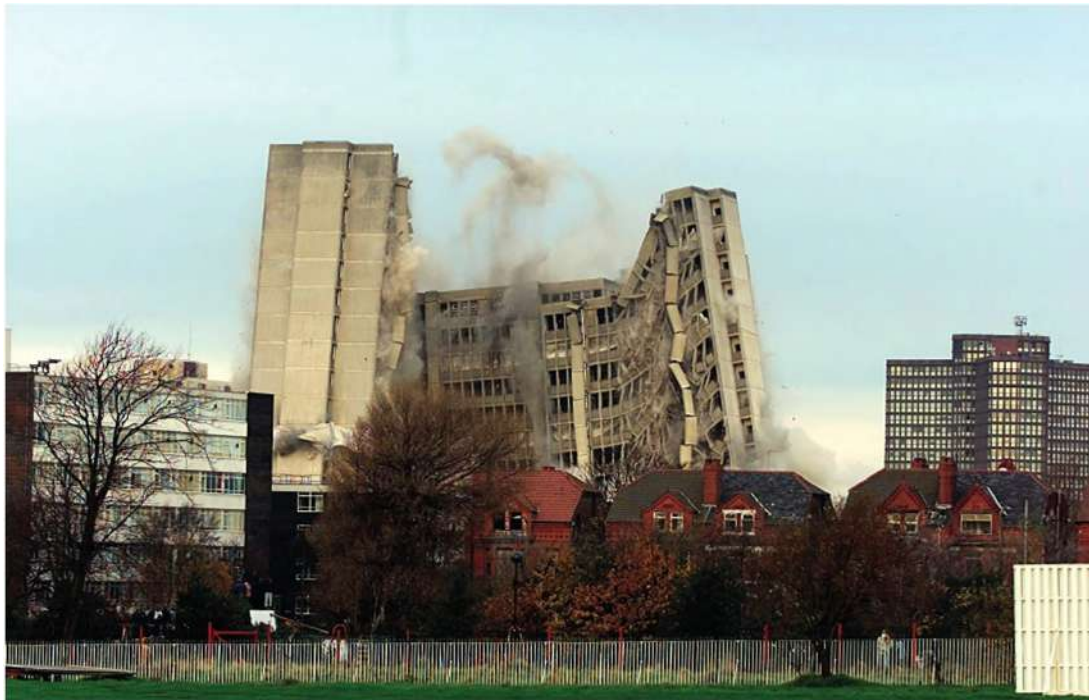
Figure 6.12: The demolition of an old housing estate in Liverpool
