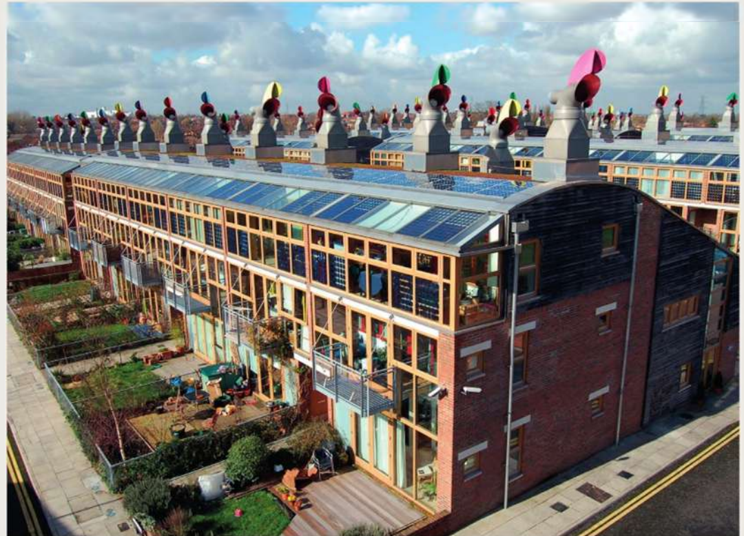
Figure 6.25: BedZED, a zero-energy urban development
