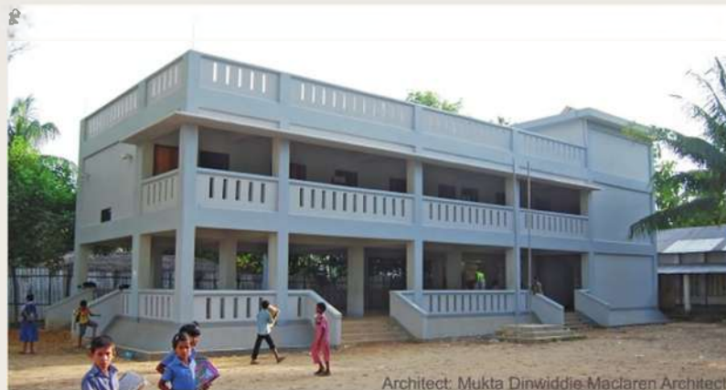
Figure 3.34: A multipurpose cyclone shelter at Chittagong, Bangladesh, with solar power, rainwater harvesting and first-aid room – built with US government funding to withstand strong earthquakes and 260 km/h winds
