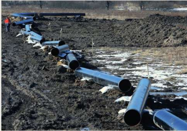
Figure 2.36: Gas pipeline construction in Russia
