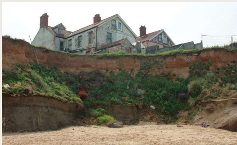
Figure 6.17: Houses in Happisburgh nearing the cliff edge, 2010 (now demolished as part of the Pathfinder Pilot Project)
