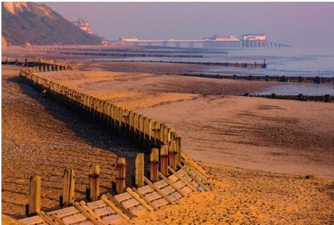
Figure 3.32: Examples of hard engineering – revetments and groynes at Overstrand, Norfolk
